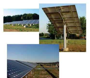
Our project will have panels between 2.5 metres and 4 metres high. The panels will be mounted on fixed-axis racks oriented in rows spaced up to 10 metres apart.
